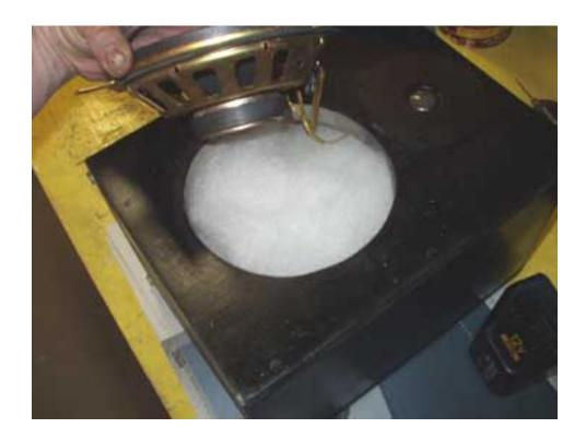
Install the tweeter and midrange driver using #6 x ¾" screws, and pre-drill your holes. At this time, complete your grille construction as described in the previous article and install. As you make the final wiring connections, keep in mind the polarities. Before you install the grilles, you might want to hook the speakers up for a final listening test.
